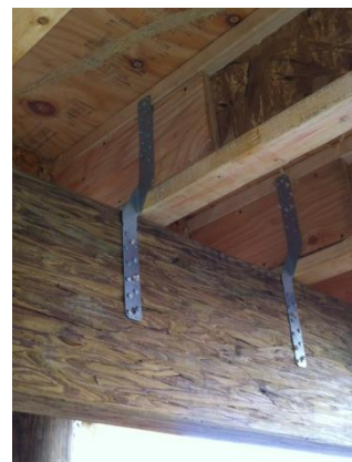
Figure 8: Joist to Beam Connection Detail.
