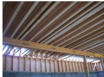
*The in-field substitution of lower-design value I-joists in this custom home required the costly addition of a beam and support columns, and potentially disappointed homeowners from the loss of clear space in this room.*
