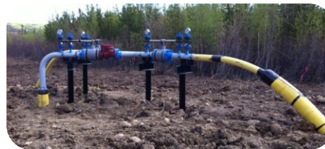
Pipeline construction in Saddle Hills, Alberta
