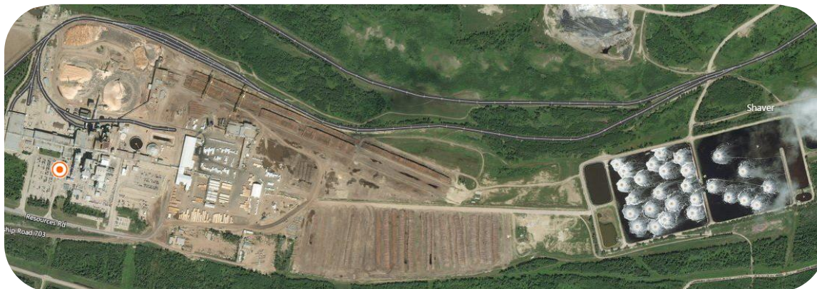
Weyerhaeuser and International Paper facilities in Grande Prairie, Alberta
