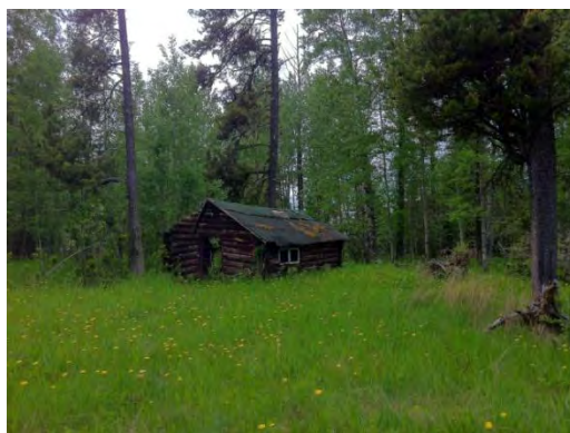
Intact Trapper Cabin
